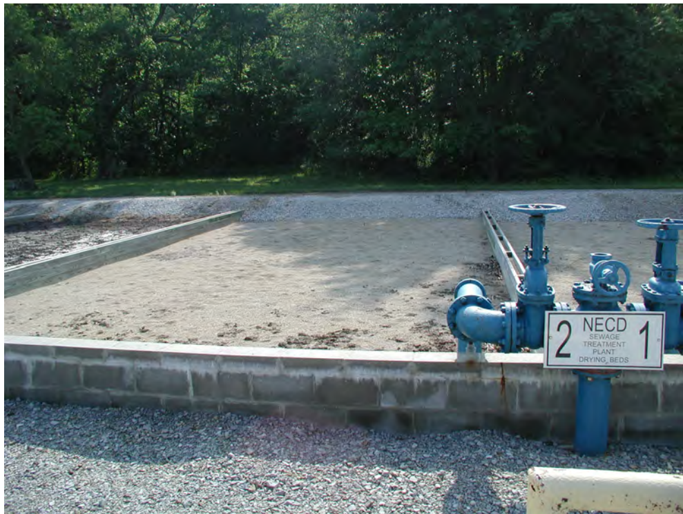
Photograph 121. STP Sludge Bed
