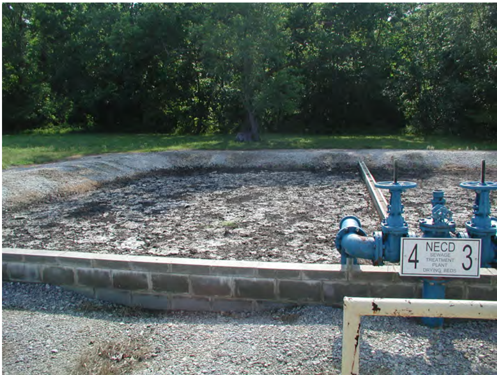
Photograph 123. STP Sludge Bed
