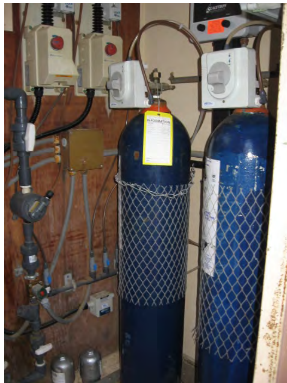
Photograph 119. STP – sulfur dioxide and chlorine tanks
