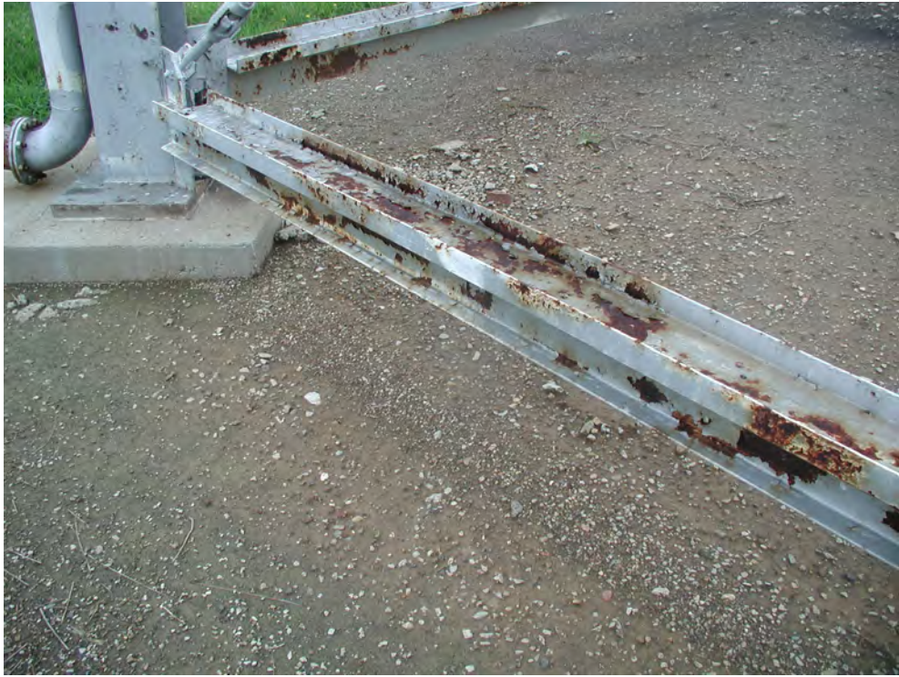
Photograph 134. Structure 510 – Flaking Paint
