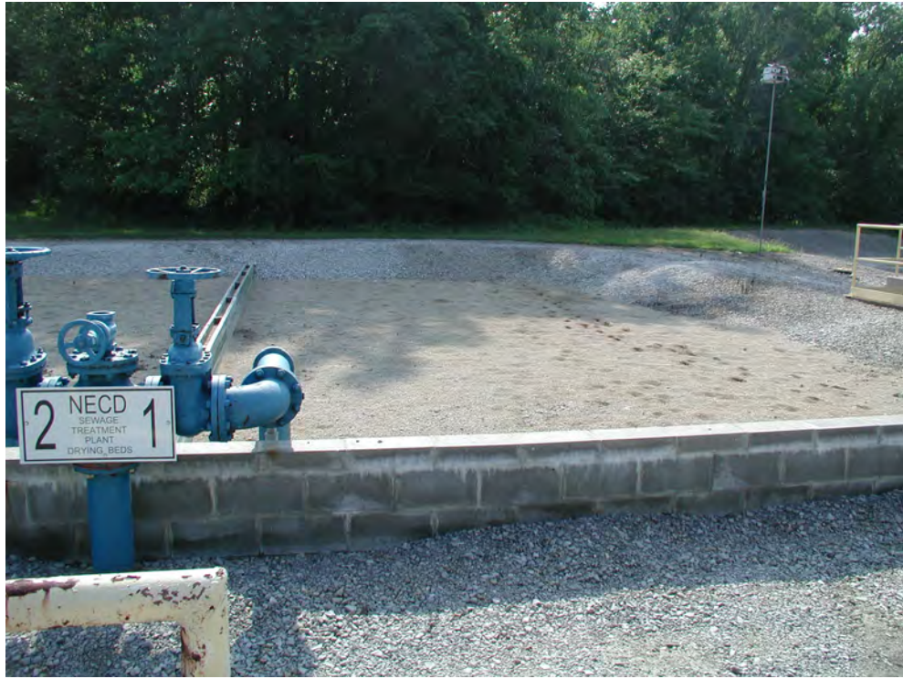
Photograph 120. STP Sludge Bed
