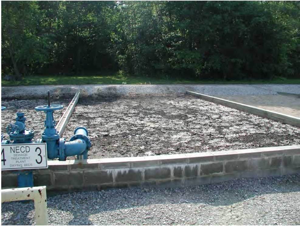
Photograph 122. STP Sludge Bed
