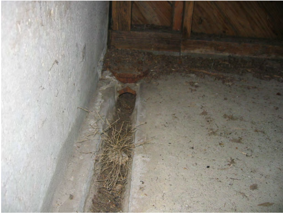
Photograph 55. Interior of Richmond Magazine 50 – floor gutter leading to exterior of building
