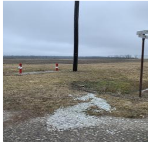
Photo 20. Photo of hydrants.
