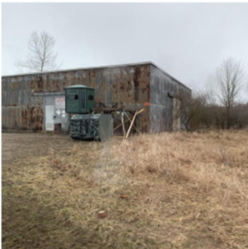
Photo 47. Photo of former hazardous waste storage building.
