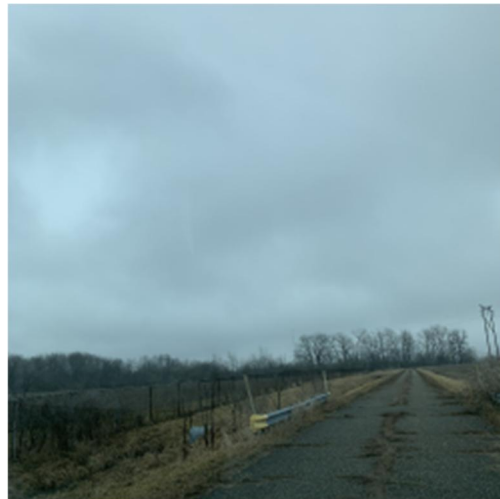
Photo 40. Photo of the site looking east.
