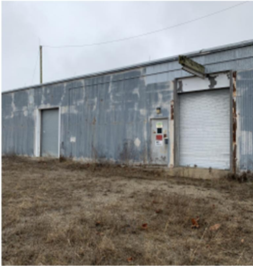
Photo 49. Photo of former hazardous waste storage building.
