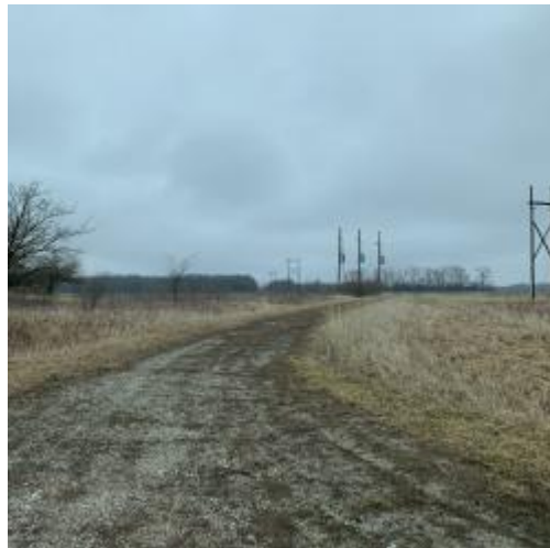
Photo 30. Photo of pole mounted transformers.
