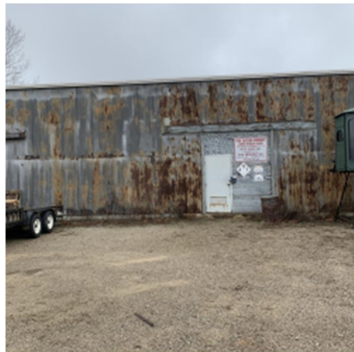
Photo 46. Photo of former hazardous waste storage building.
