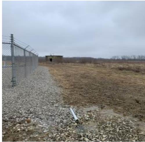
Photo 26. Photo of outbuilding looking east.
