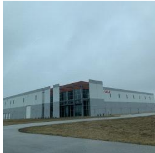
Photo 2. Photo of shell building looking northwest.
