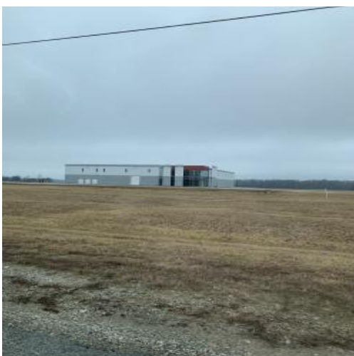
Photo 17. Photo of site looking northeast.
