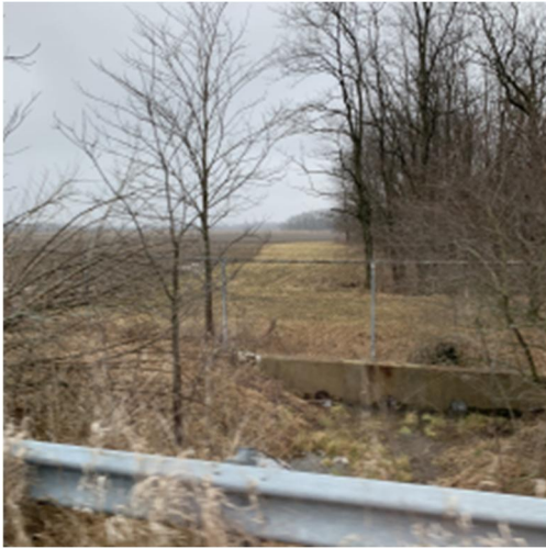
Photo 43. Photo of the drainage culvert.
