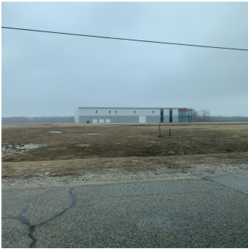
Photo 1. Photo of shell building looking north.
