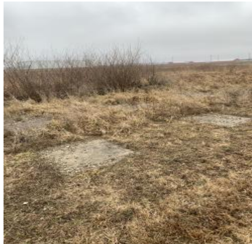
Photo 28. Phot of concrete pads.
