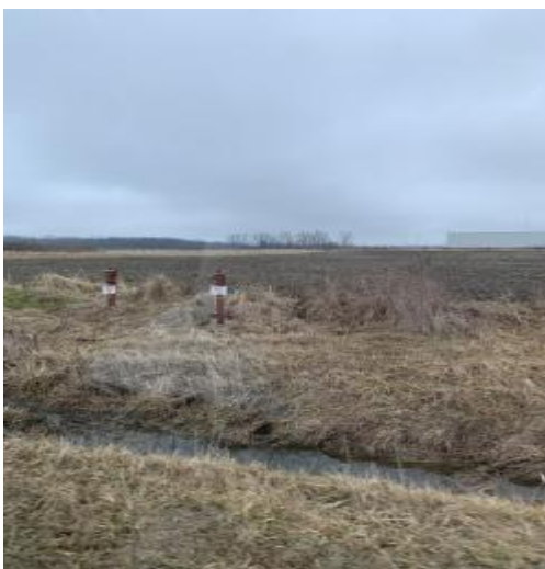
Photo 23. Photo of hydrants.
