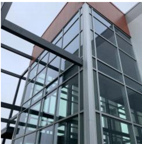
Photo 5. Photo of front entry of the shell building.
